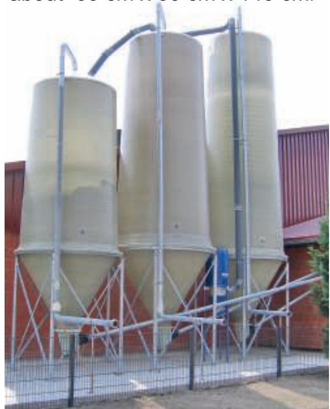
AirCleaner with connection to three silos and outlet pipe into feeding system
