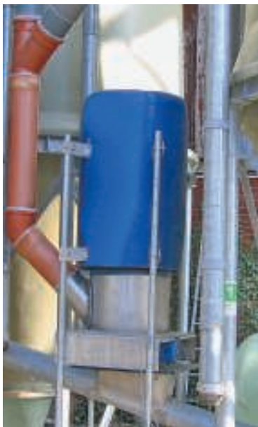
AirCleaner with connection to three silos and outlet pipe into feeding system
